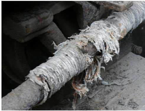
Hot water pipes wrapped in friable woven ACM textile
