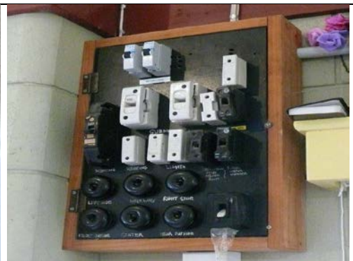
Cement sheet (black) switch backing
