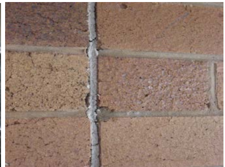
ACM as joint sealant
