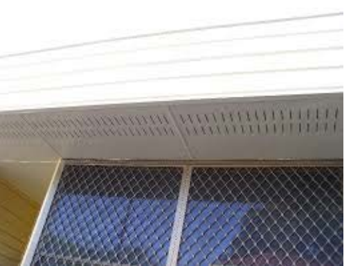
Slotted soffit cement sheet eave
