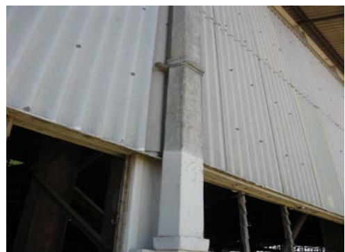
Square ACM downpipe
