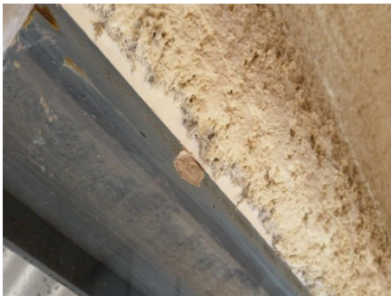
Spray-on cement ceiling render
