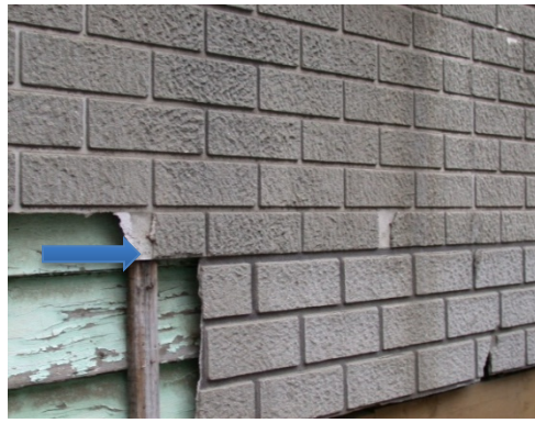
False brick cladding
