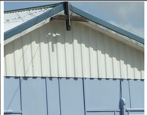
"Shadowline" cement sheet gable
