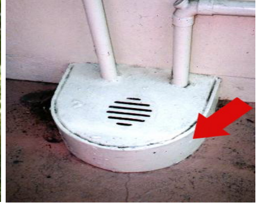
Drain trap surround
