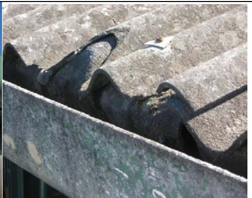
Gutter and roof
