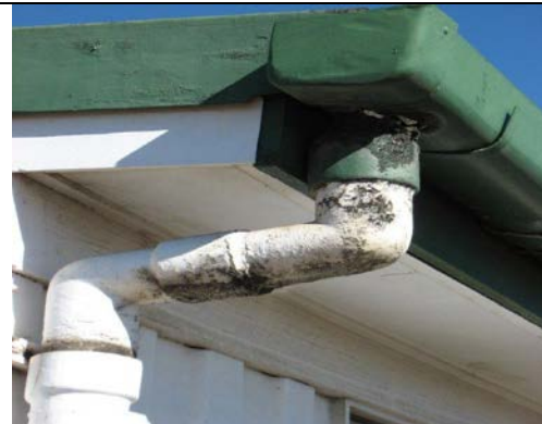
Gutter and downpipe
