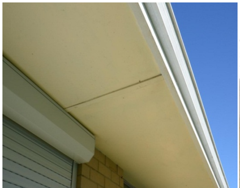
Cement sheet eave
